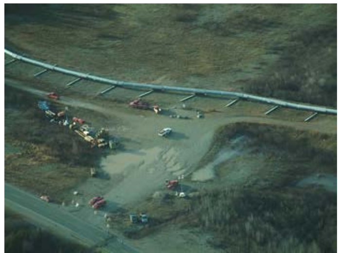
Figure EQ.54 Map showing location of 2 earthquakes occurring in Alaska in October-November 2002. Photo on right shows the Trans-Alaska Pipeline running parallel to the fault. Note the rails supporting the pipeline.
