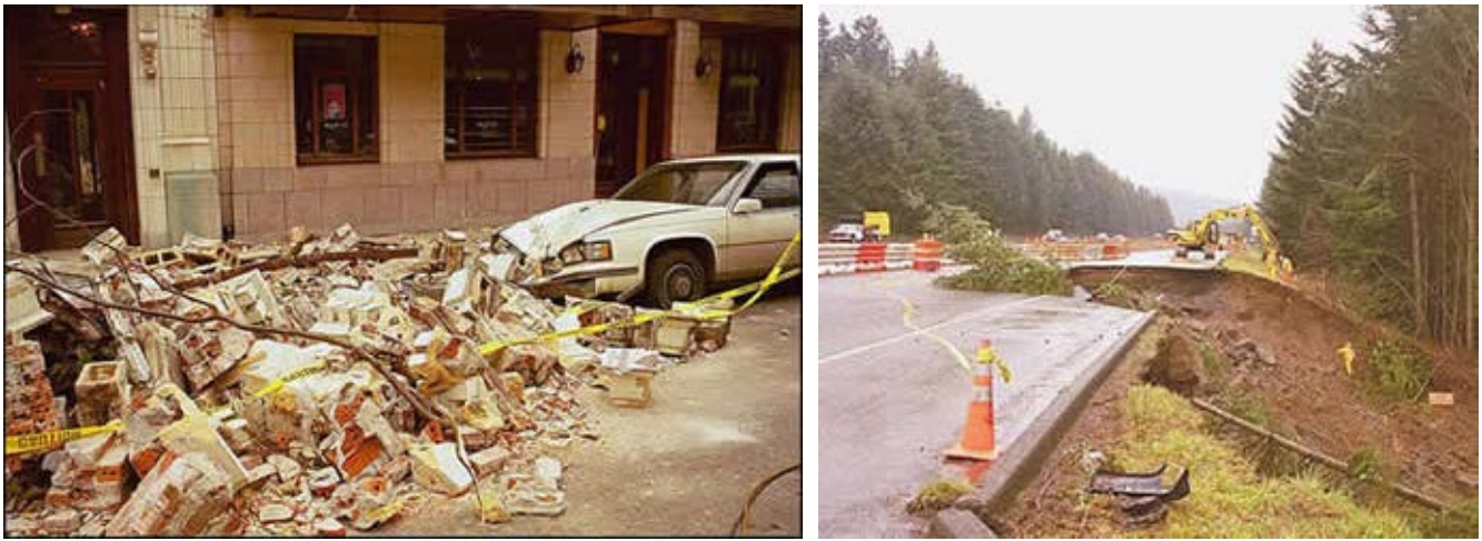
Figure EQ.11 Images of damage to buildings and cars near the Washington Capitol Building in Olympia, WA (left) and to Highway 101 (right). Photos retrieved from The Nisqually Earthquake Information Clearinghouse.
