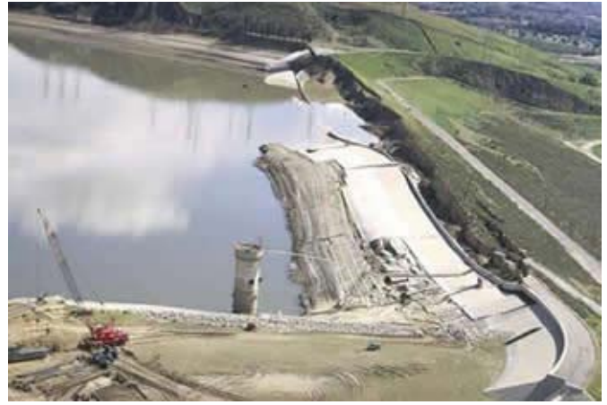
Figure EQ.66 (Left panel) Photo of buildings that were destroyed because of liquefaction following an earthquake near Niigata, Japan, 1964. (Right panel) Photo of an earth dam that was very nearly breached (water breaking through) as a result of liquefaction caused by earthquake shaking. Less than a minute more of shaking and the valley below would have been devastated.
