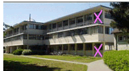
Figure EQ.63 (Top panel) Damage to a building with a "soft" storey. (Right panel) Examples of how selected buildings on UBC campus have been strengthened (braces are highlighted in magenta).
