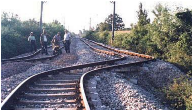
Figure EQ.16 (Left panel) A displaced a railway line caused by a strike-slip fault rupture following the earthquake in Izmit, Turkey, on August 17, 1999. (Right panel) Rupture caused by movement on the Fault near the city of Bam, Iran.
