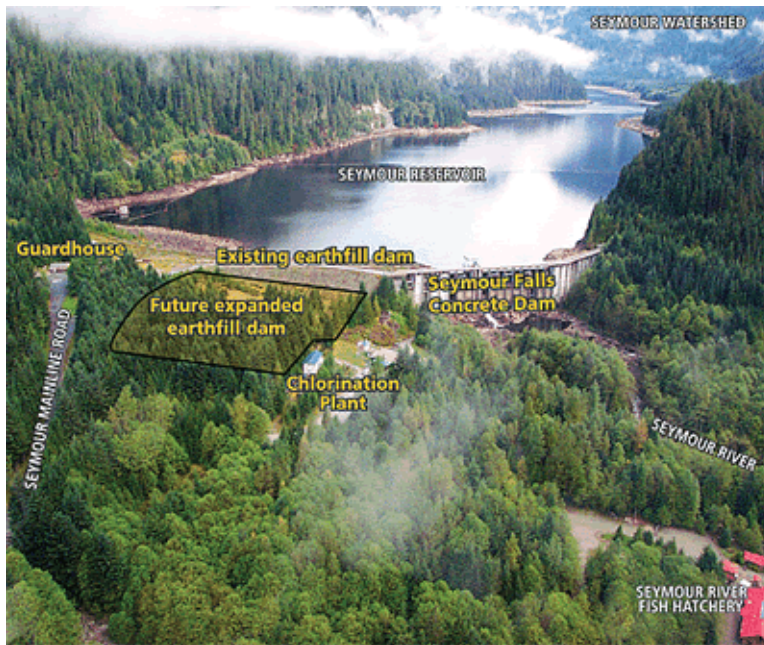
Figure EQ.61 Seymour Falls and the planned upgrades projected for completion by 2007. The upgrades will ensure that the Dam performs safely in the event of a major earthquake. Photo from Metro Vancouver.
