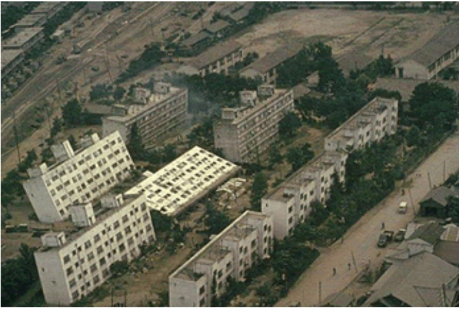
Figure EQ.66 (Left panel) Photo of buildings that were destroyed because of liquefaction following an earthquake near Niigata, Japan, 1964. (Right panel) Photo of an earth dam that was very nearly breached (water breaking through) as a result of liquefaction caused by earthquake shaking. Less than a minute more of shaking and the valley below would have been devastated.
