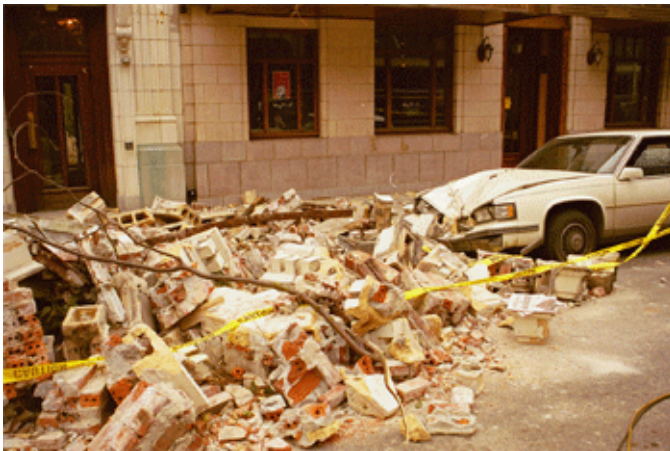
Figure EQ.64 (Top left panel) Bricks that fell because they were not properly attached to a building near the Washington Capitol Building in Olympia, WA causing damage to cars and other properties on the ground. Photo retrieved from the U.S. Geological Survey and The Nisqually Earthquake Information Clearing House (Top right panel) Concrete failure at the join between two sections of reinforcing, Interstate 880 in California. (Bottom right panel) Slope damage near a home following a landslide caused by an earthquake.
